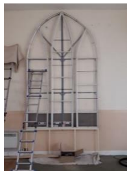
The various stages of the window's reconstruction in the church
